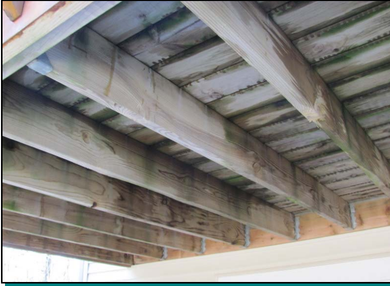
Wood balcony framing
