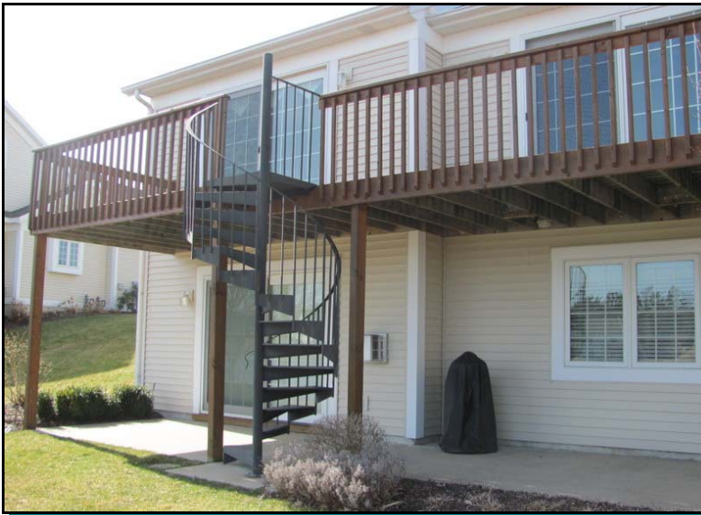
Metal spiral staircase at rear balcony
