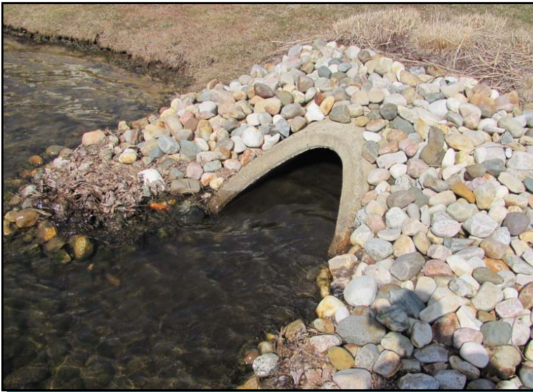
Concrete drainage structure
