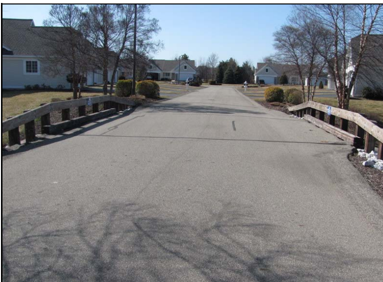
Asphalt pavement overview at Timber Crossing bridge
