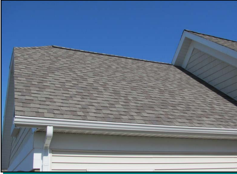
Asphalt shingle roof
