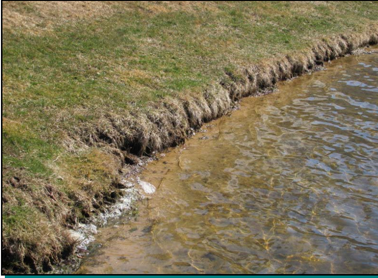
Minor shoreline erosion
