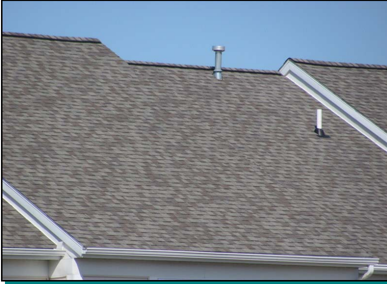
Asphalt shingle roof overview
