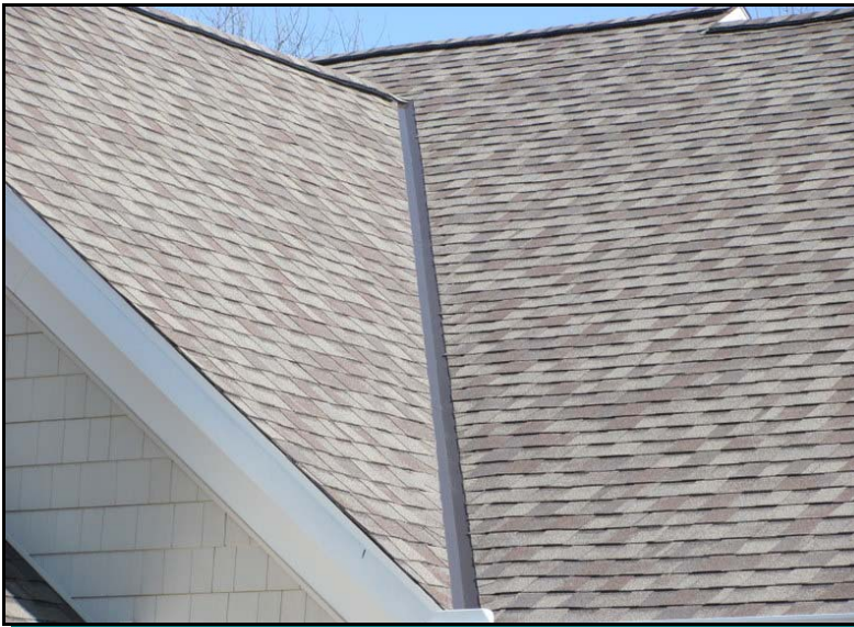
Valley flashing at roof
