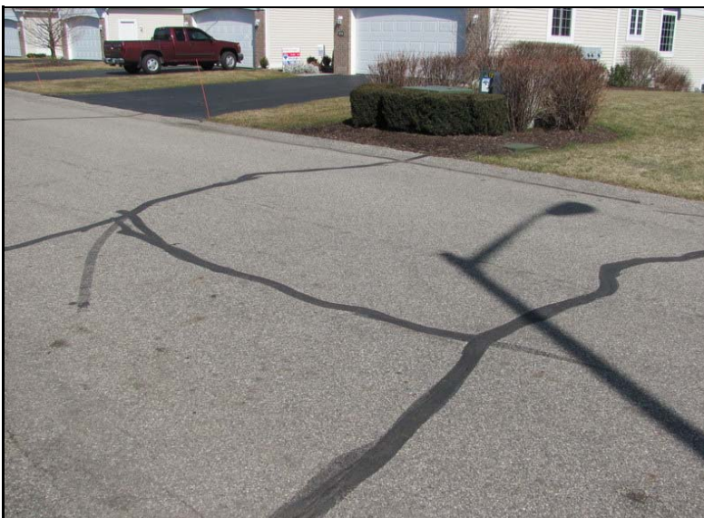
Longitudinal and transverse crack repair
