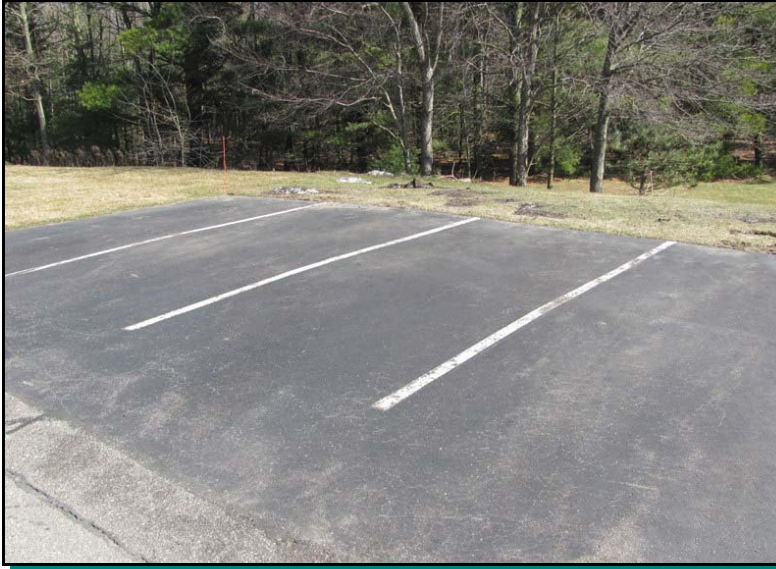
Asphalt parking area
