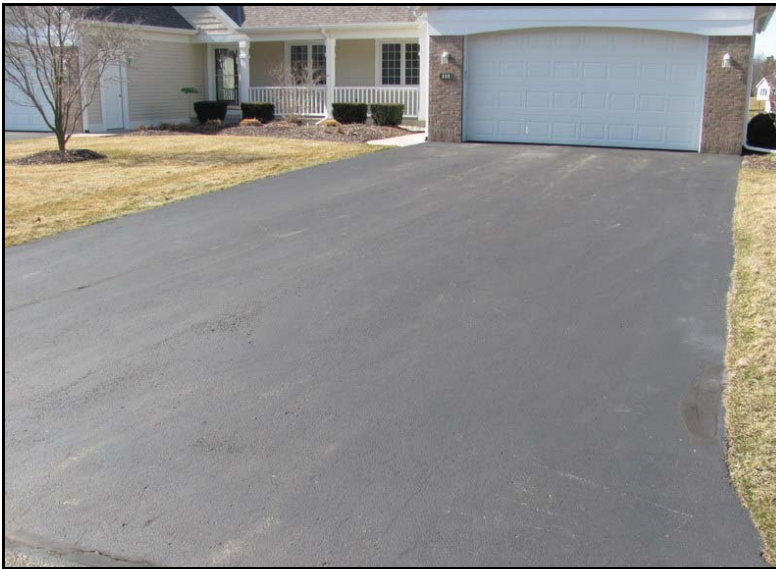
Asphalt driveway overview
