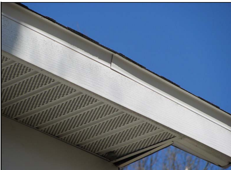
Drip edge flashing at roof
